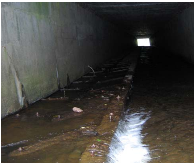
Photo: Baffle system in a Sucker River box culvert, under Highway 61.
