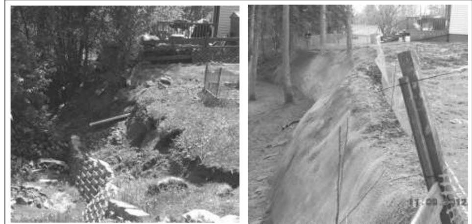
A 'before' photo (L) shows part of the severe bank failure near two homes above Chester Creek, where saturated soils caused a block retaining wall to slump. After (R), shows emergency bank stabilization applied to the edge of both properties, using a technique called 'soil nailing'.
