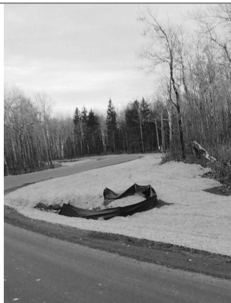
Before, at left, erosion beginning along the side of this development driveway; at right, proper grading, mats and barriers stabilize soils until vegetation takes root.
